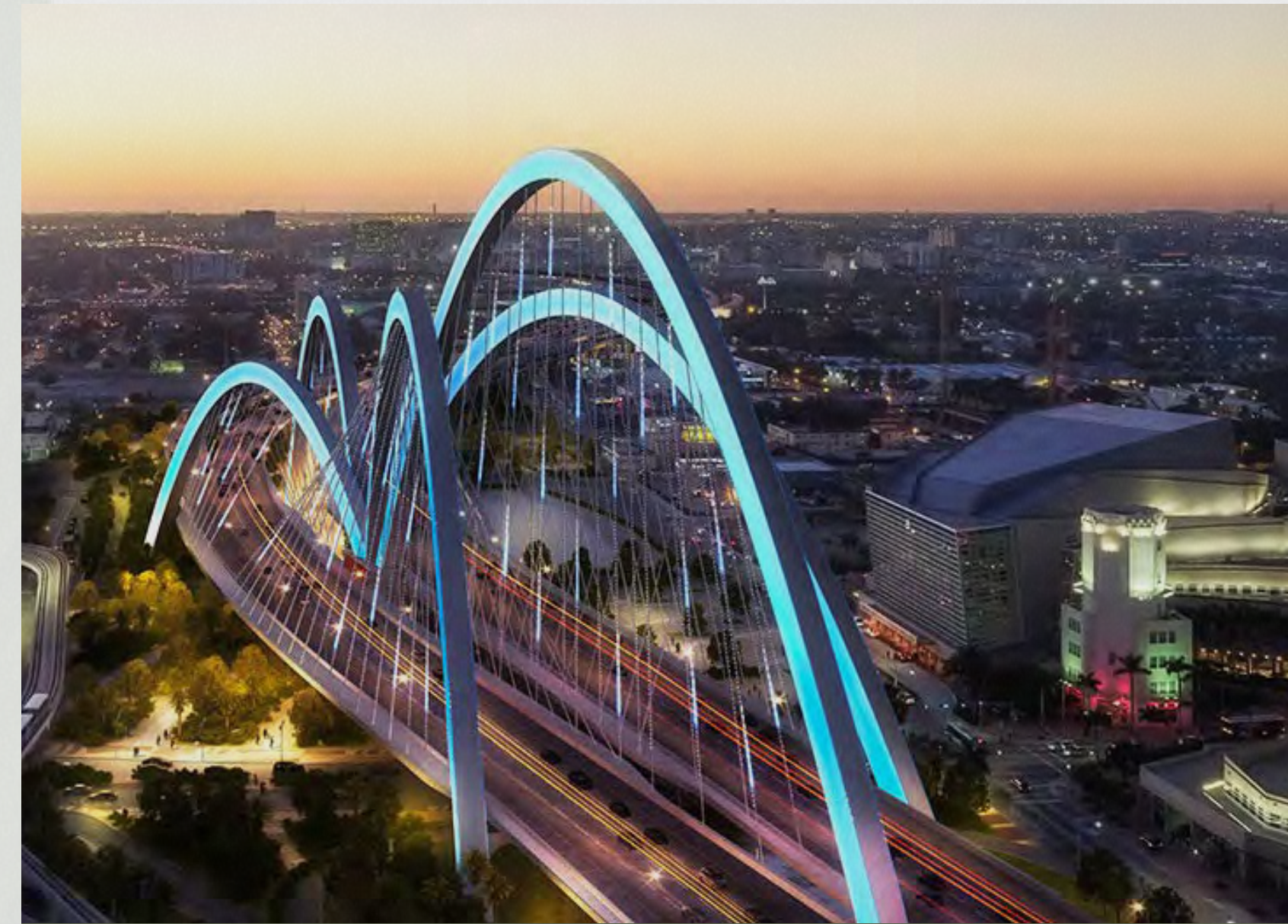
I-395 SIGNATURE BRIDGE
